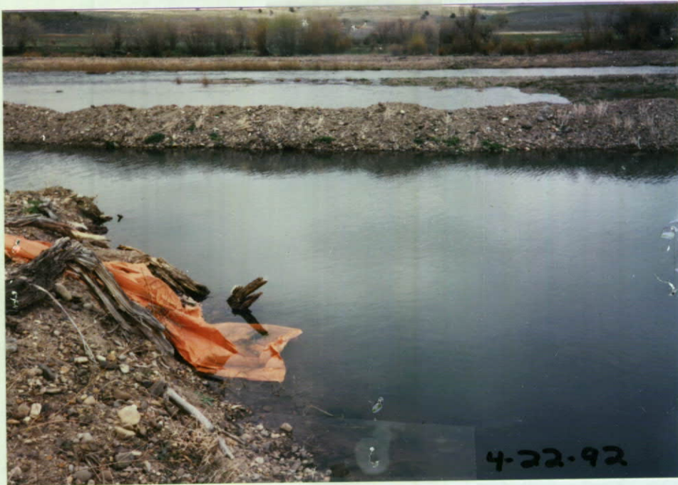
Diversion from Jordan creek.
