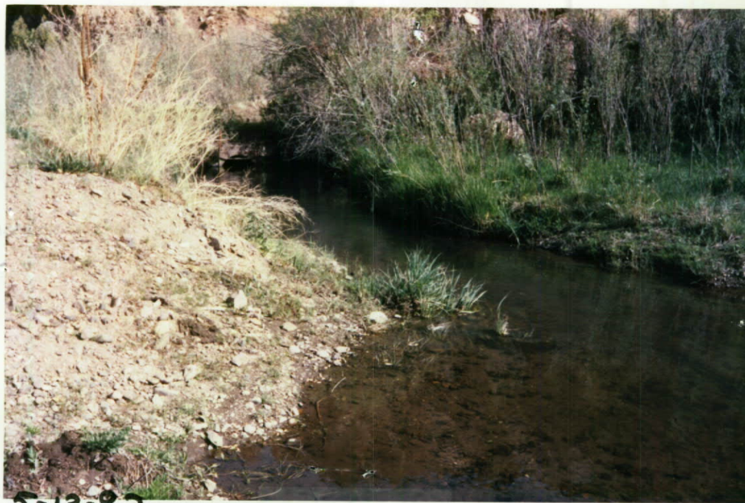
Diversion in Sec. 19, S&NW. Conveyed by ditch. 36" culvert
