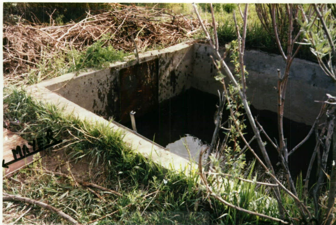
Headgate where ditch splits & takes water to Bruce & Mayer.
