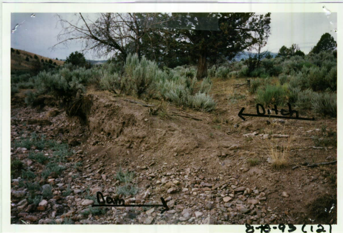
Diversion no. 2, gravel & rock dam & ditch to place of use.
