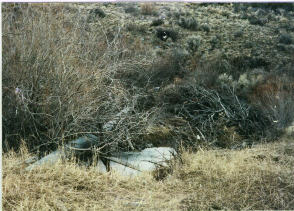
Where pipe crosses creek from ditch to irrigate field south of creek.
