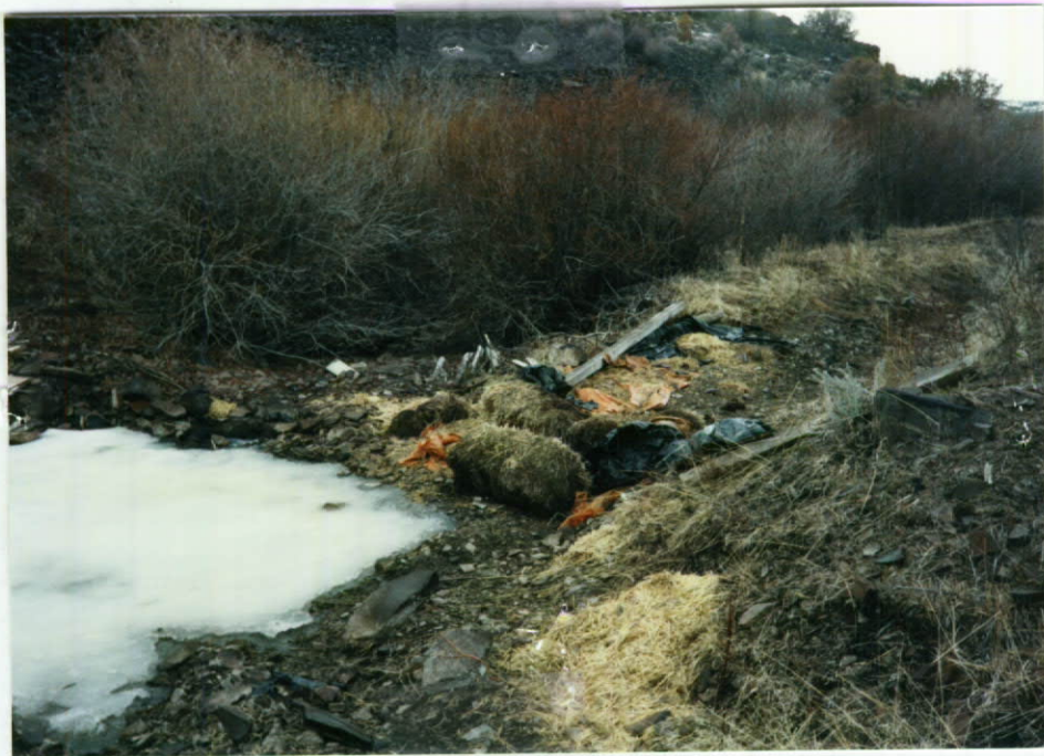
Diversion dam located in SWNW, section 13.
