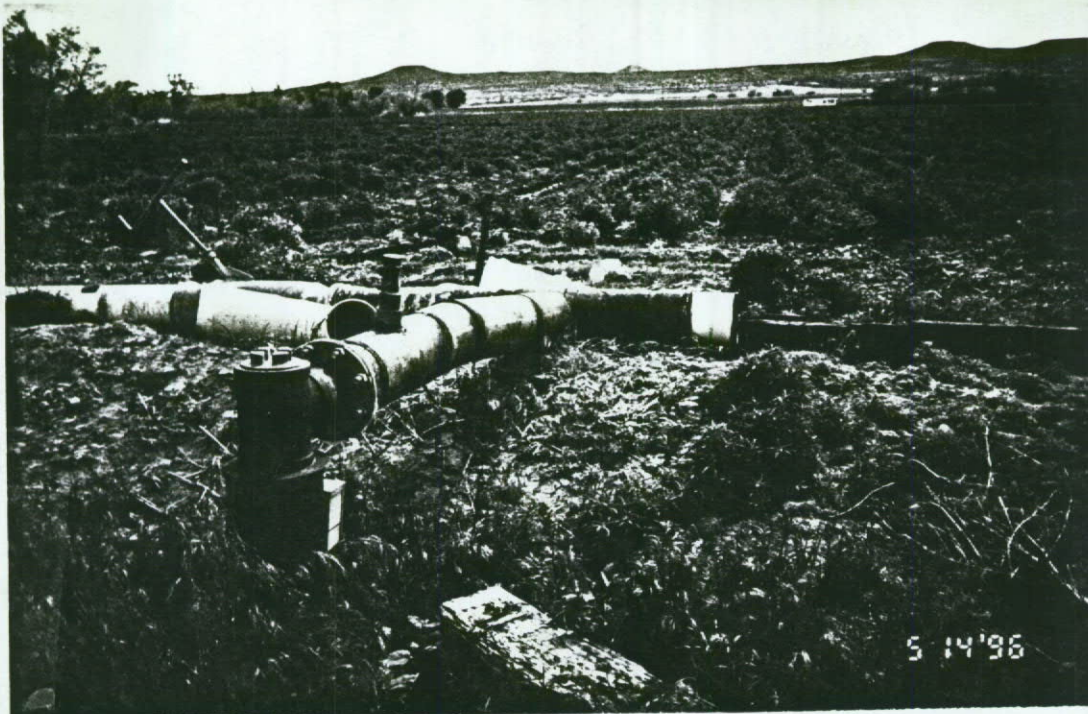
South well & P/u in NESW (view E)
