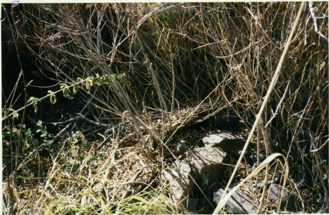
Diversion no. 1 on Cat cr., Sec. 33, NWNE
