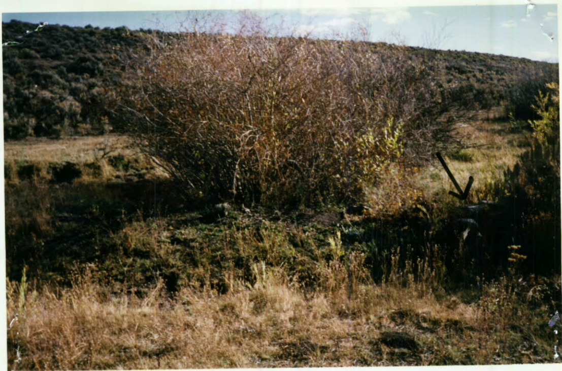
P.O.D. 1 on Alder cr. - cement culvert
