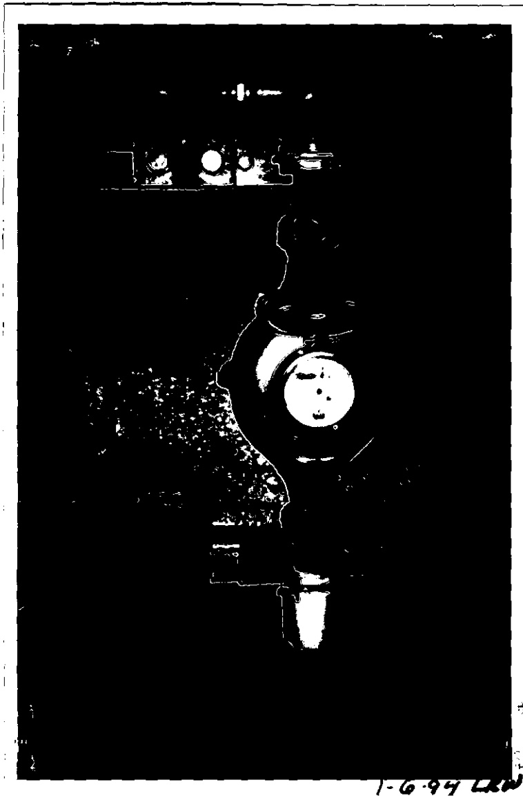
Water meter at fluoridation unit.
