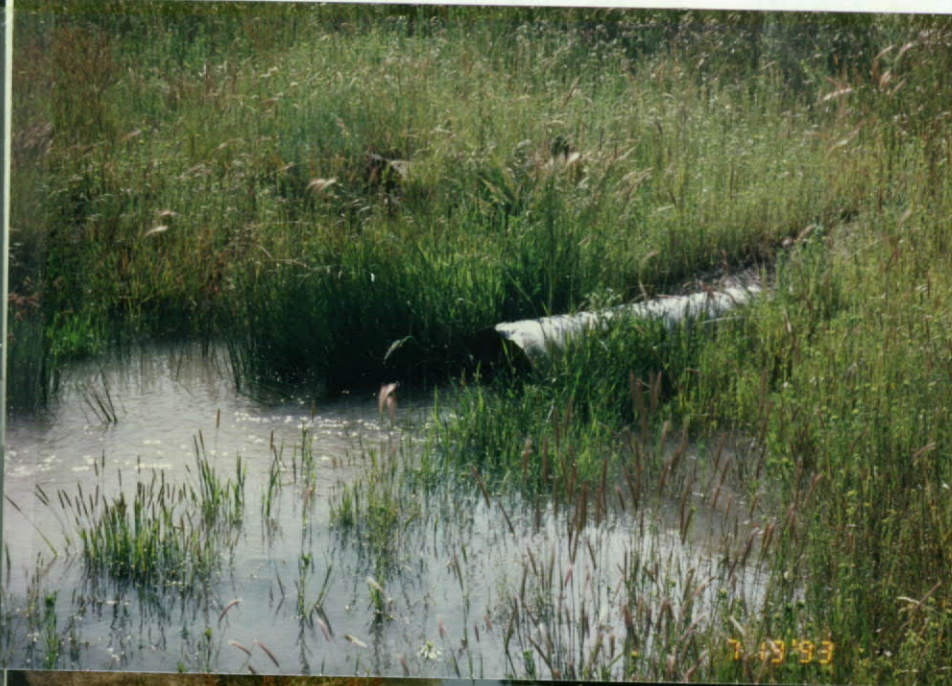
1. 15" CMP outlet pipe at the Snow Creek Reservoir, discharging.
