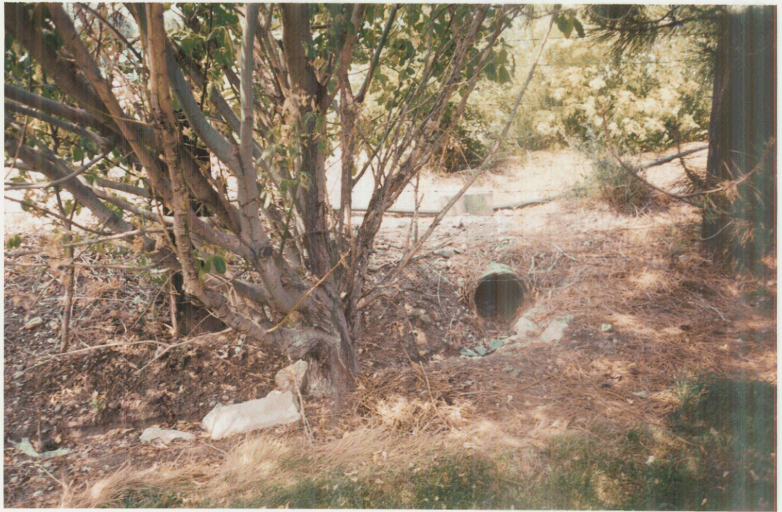
Culvert that leads to Chavers place
