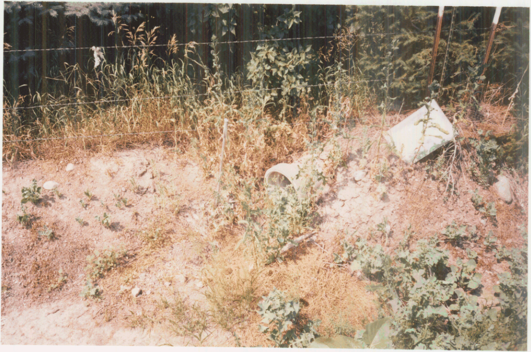
looking N. Culvert that delivers water from ditch to claimed POU.
