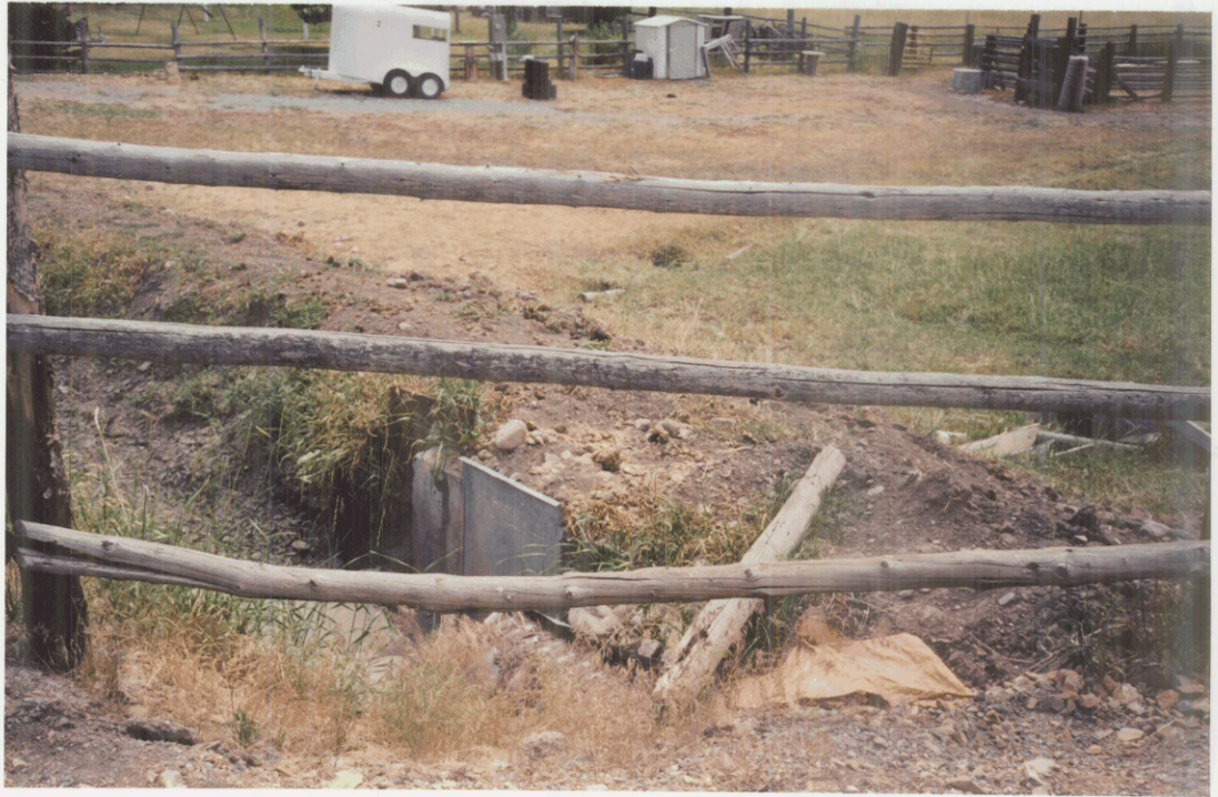
Headgate in ditch Delivery System
