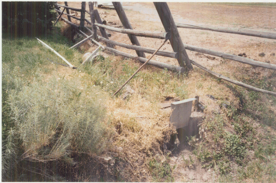
Ditch headgate - Looking West
