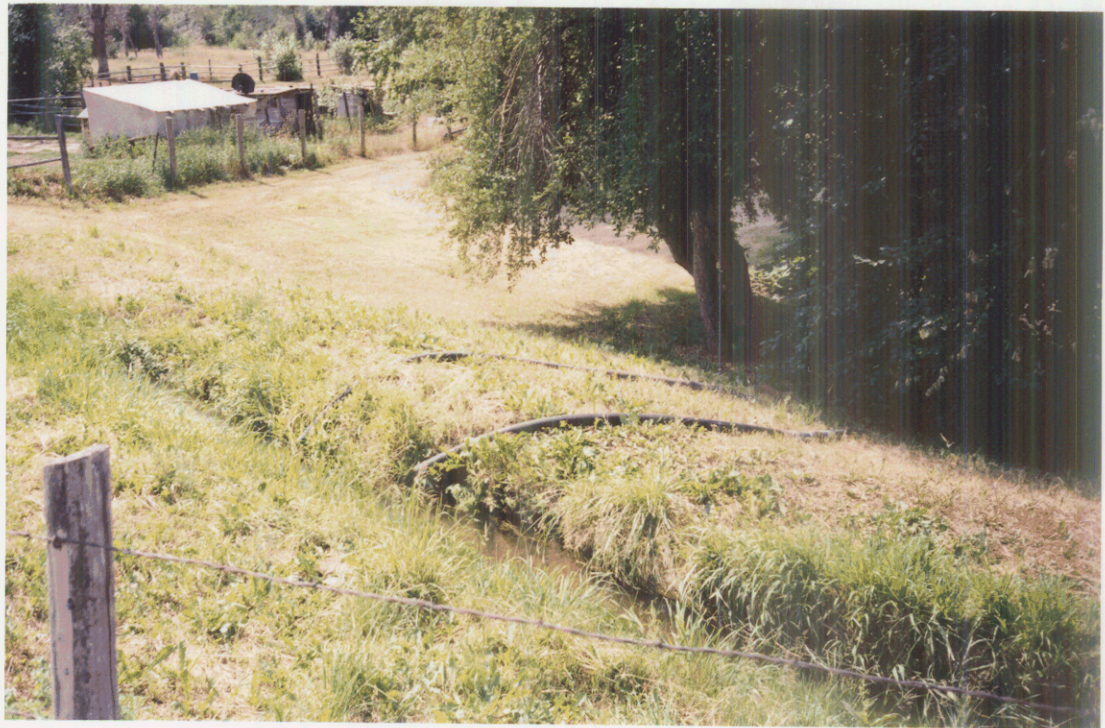
- Looking SE From N. Side of Claimant's Property. Picture Shows intake line from ditch that carries Rapid Creek water
