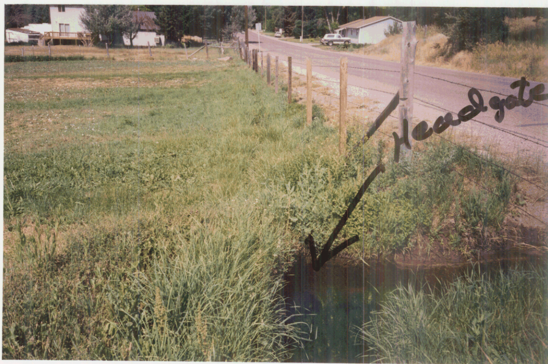
Looking W at head gate that is opened to Flood Irrigate W side of Claimed POW.
