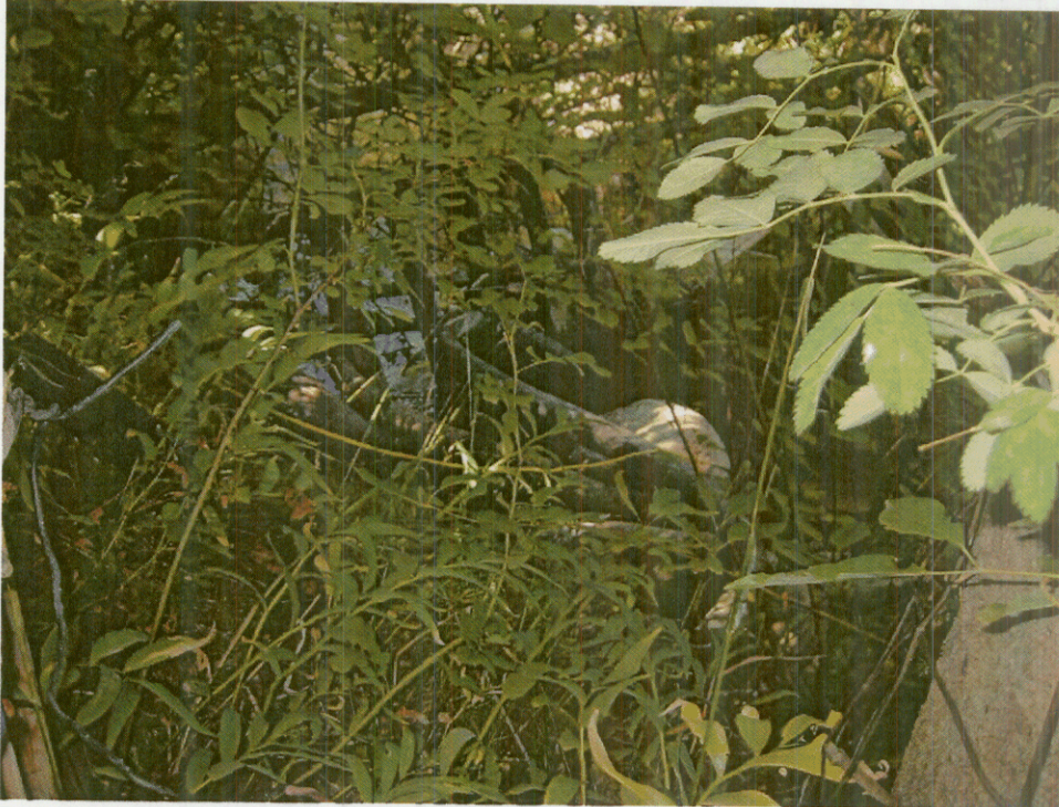
Looking South at POD. Black intake hose can be seen in picture (csaxton).
