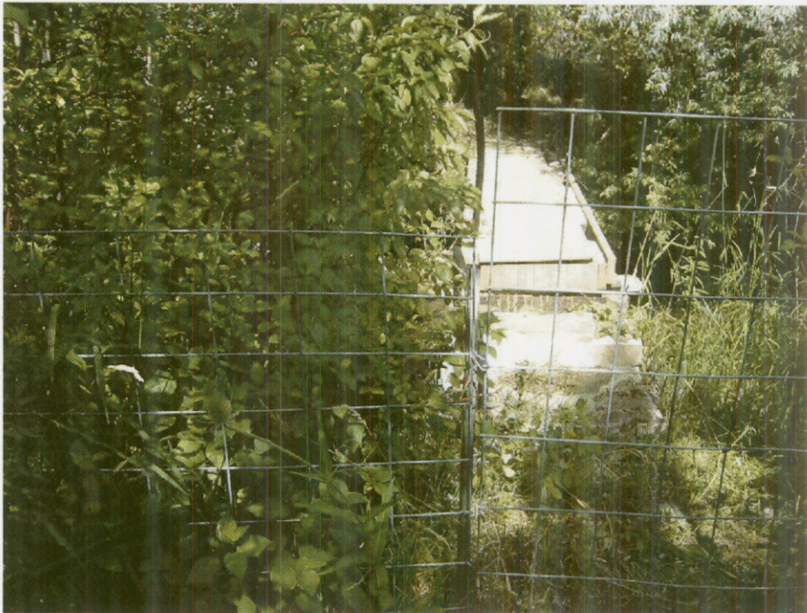
Looking East at bridge over creek. Water is diverted just North of the bridge (csaxton).
