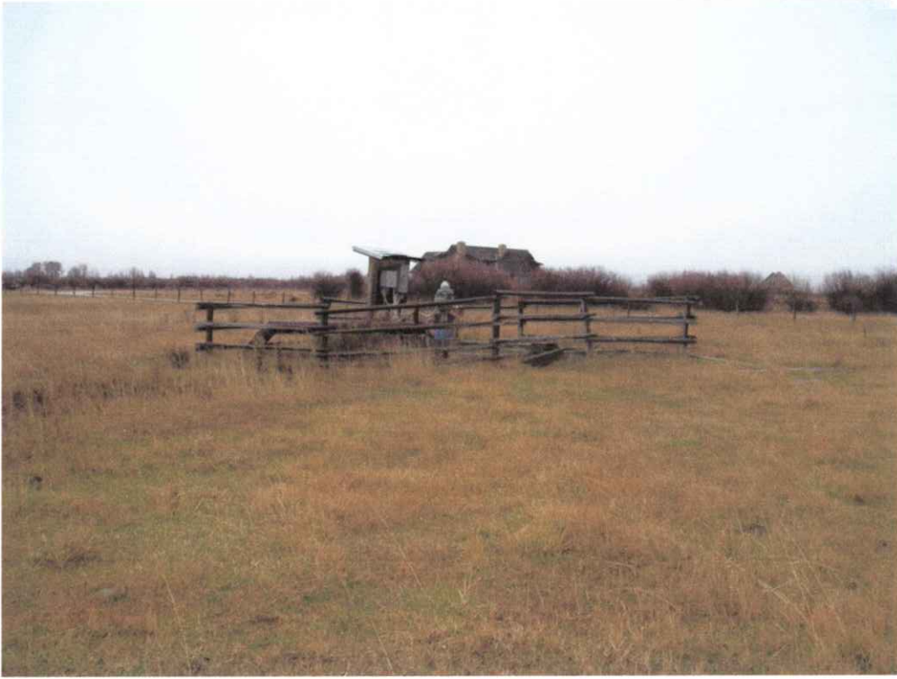
Pump on Boyd Smith diversion out of unnamed stream located near Teton River
