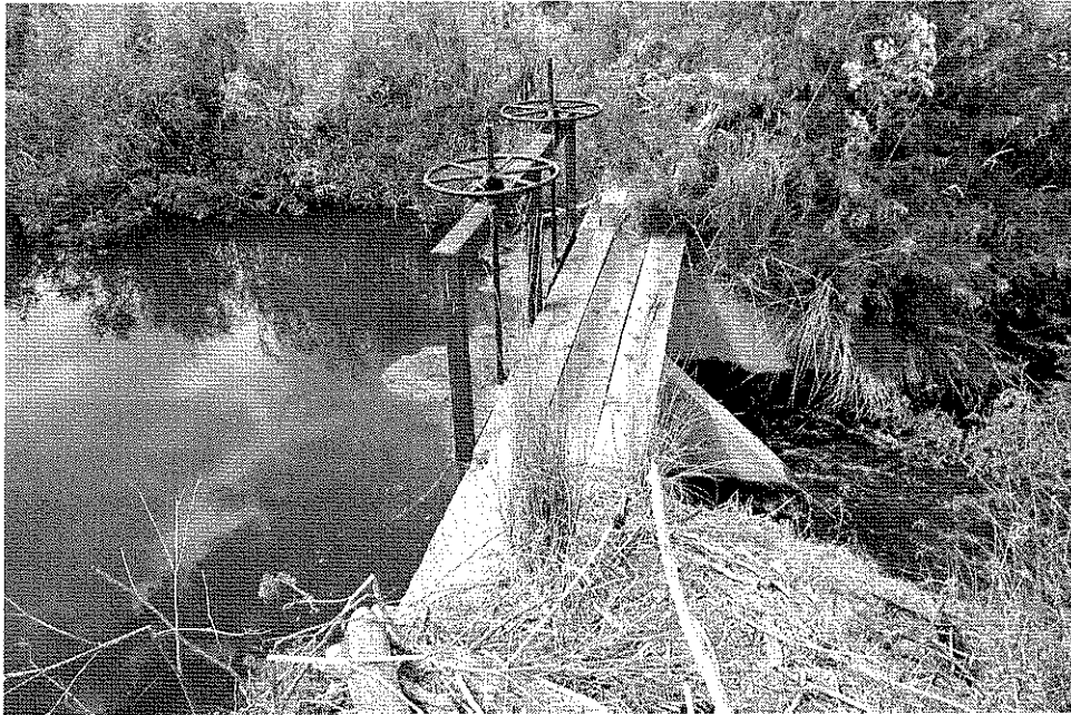
Photo 1. Johnson-Higby Ditch Headgate.
