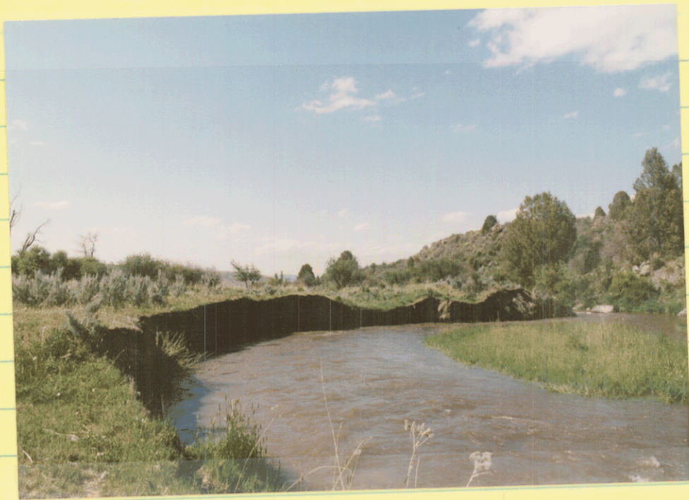
Original diversion on Bullock Place.
