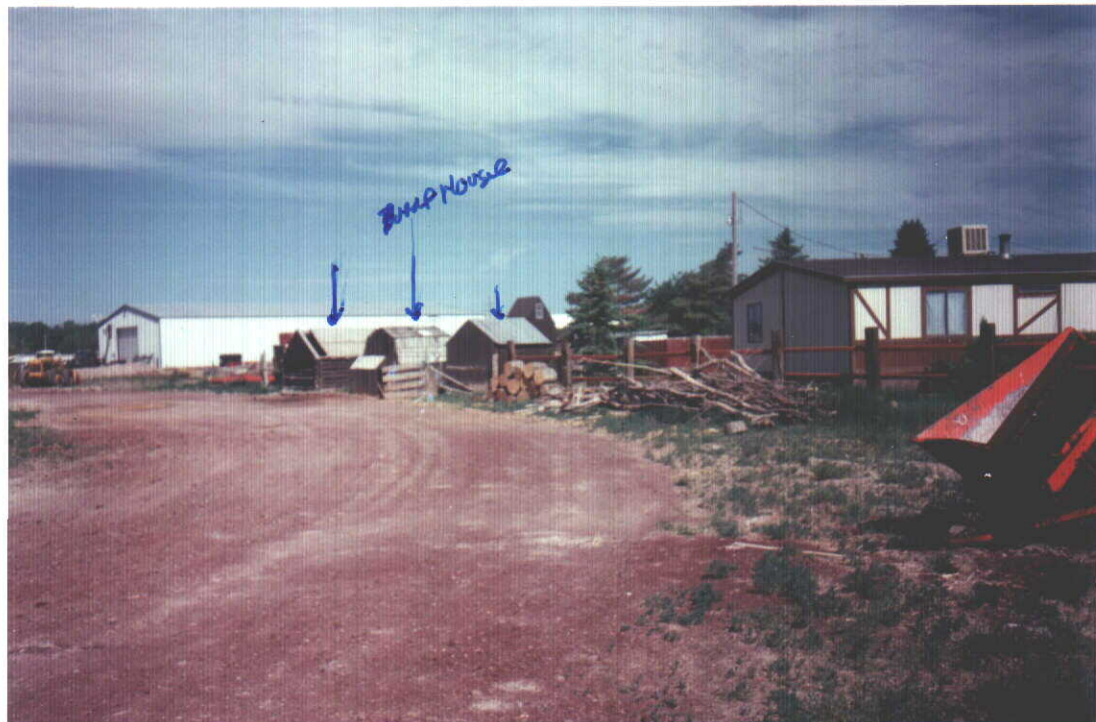
PHOTO #2 LOOKING NW TOWARDS MOBILE HOME #1 SHOWING 3 SMALL BUILDINGS. THE CENTER BLDG IS THE PUMP HOUSE.
