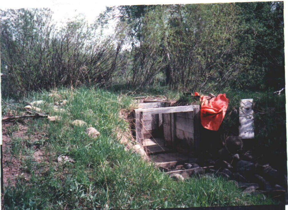
Photo #15 Diversion Box in Dry Creek Ditch - splits Ditch to Basin 21 and Basin 31
