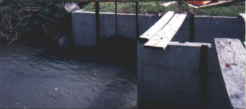
4 Foot Parshall flume at Dry Creek diversion.
