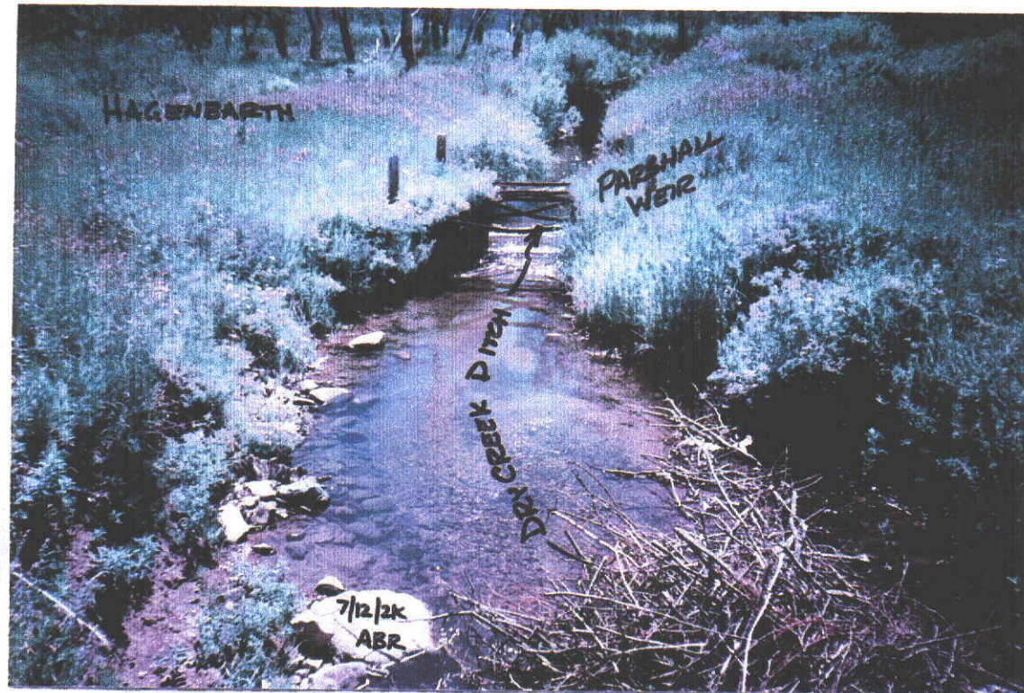
PARSHALL FLUME ON HAGENBARTH'S DRY CK DITCH.
