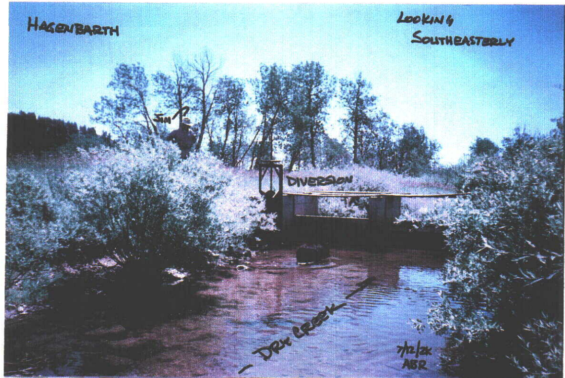
HAGENBARTH'S DRY CREEK CHECK & DIVERSION T13N R4DE SEC. 9 NE1/4SW
