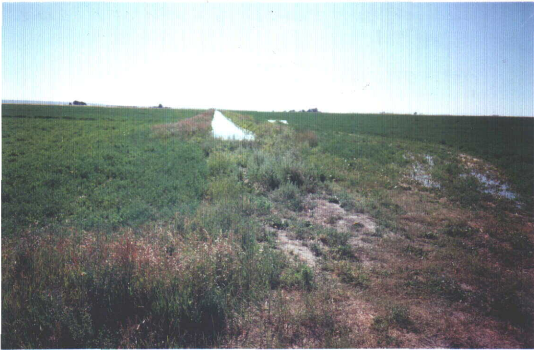
LOOKING EAST FROM 1/4 MI SOUTH OF NW CORNER,
