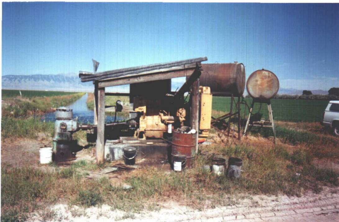
LOOKING WEST FROM 1/4 MI SOUTH OF NORTH 1/4 CORNER OF SECTION 14, APPROX. 30' EAST OF WELL,
