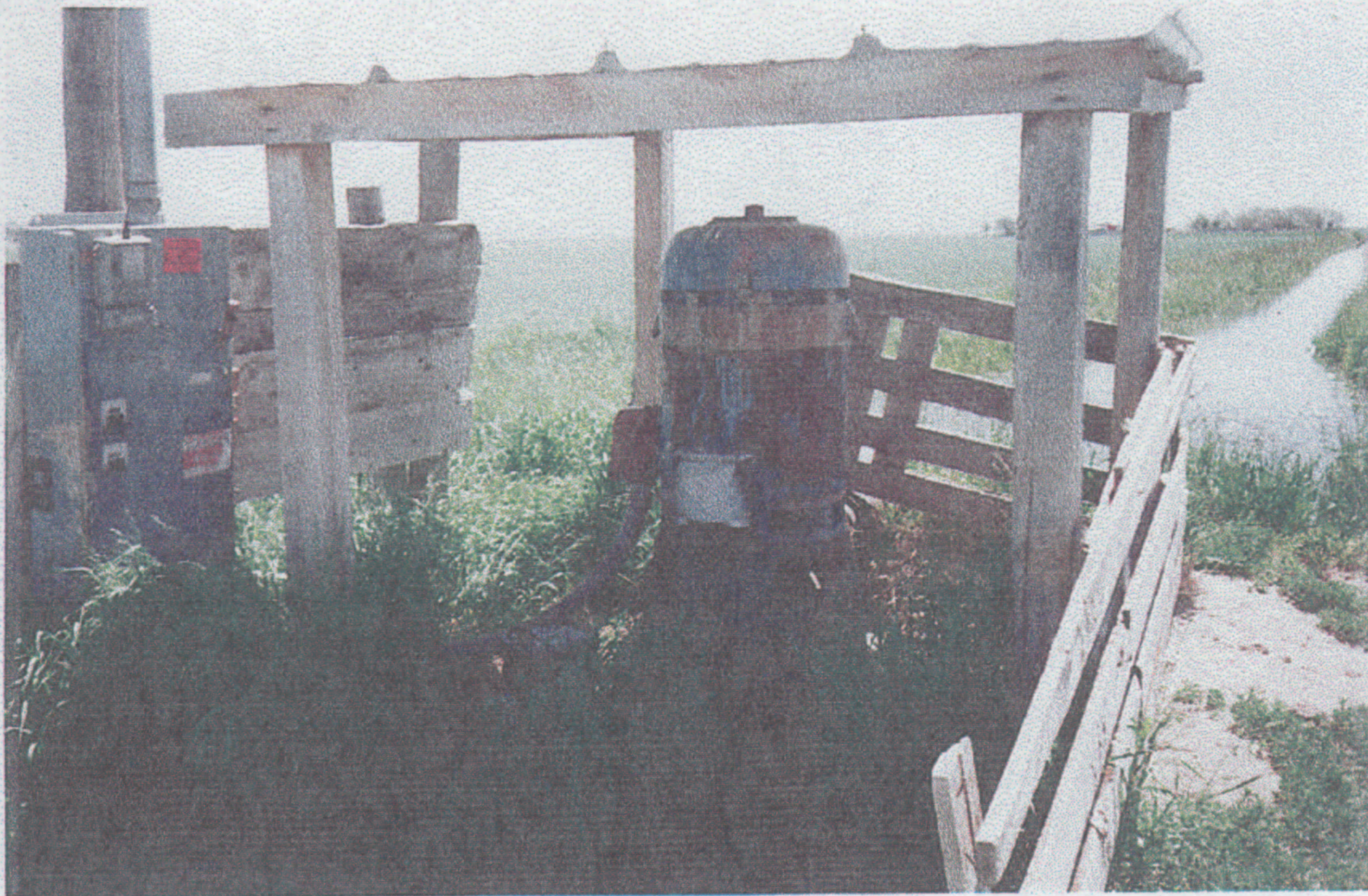
PHOTO #6 LOOKING E FROM THE CORNER OF THE SWNWNE SHOWING CAUDLE PUMP.
