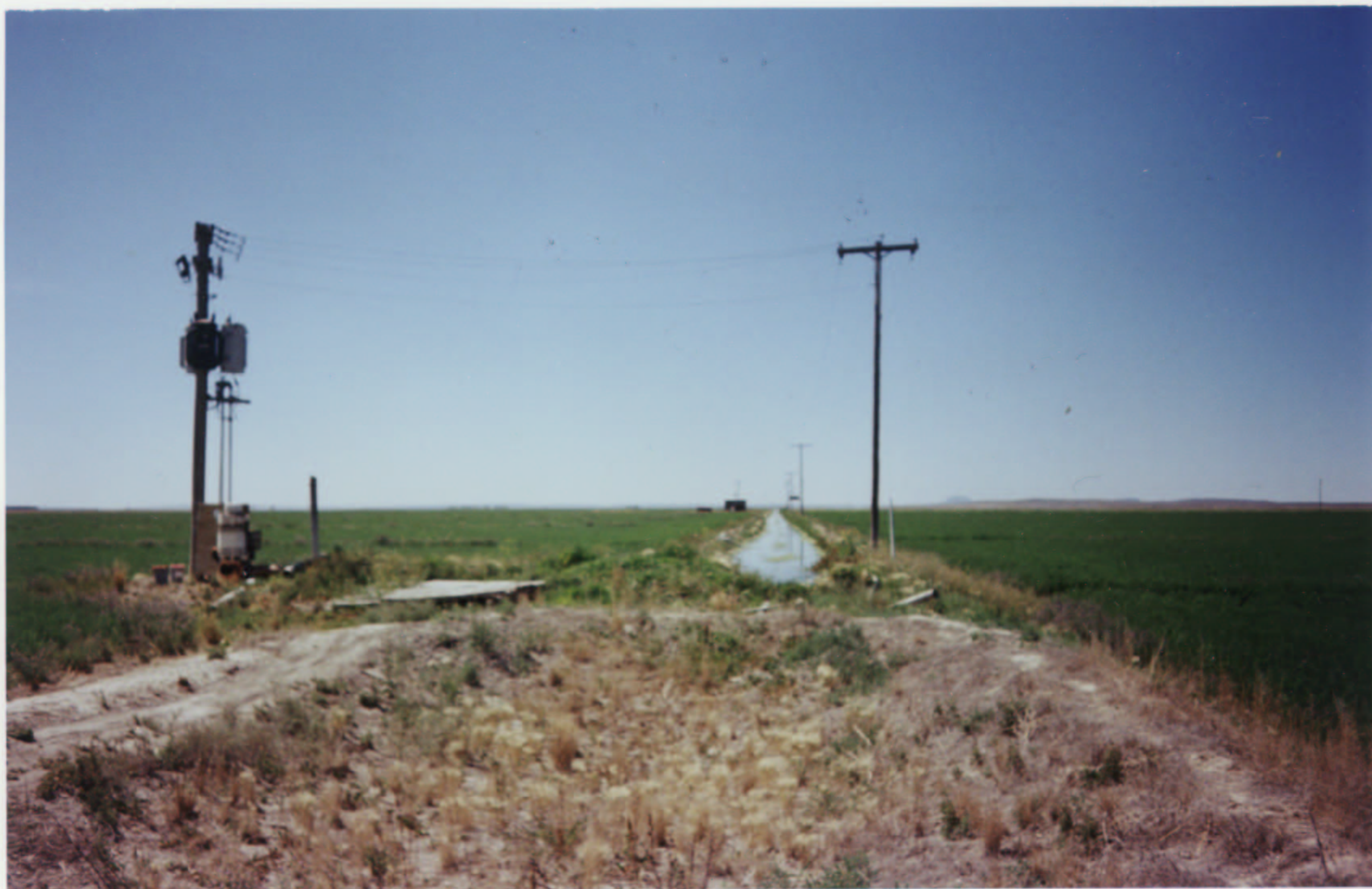
LOOKING SOUTH AT DITCH INTO WHICH THE WELLS DISCHARGE, 60' SOUTH OF COUNTY ROAD.
