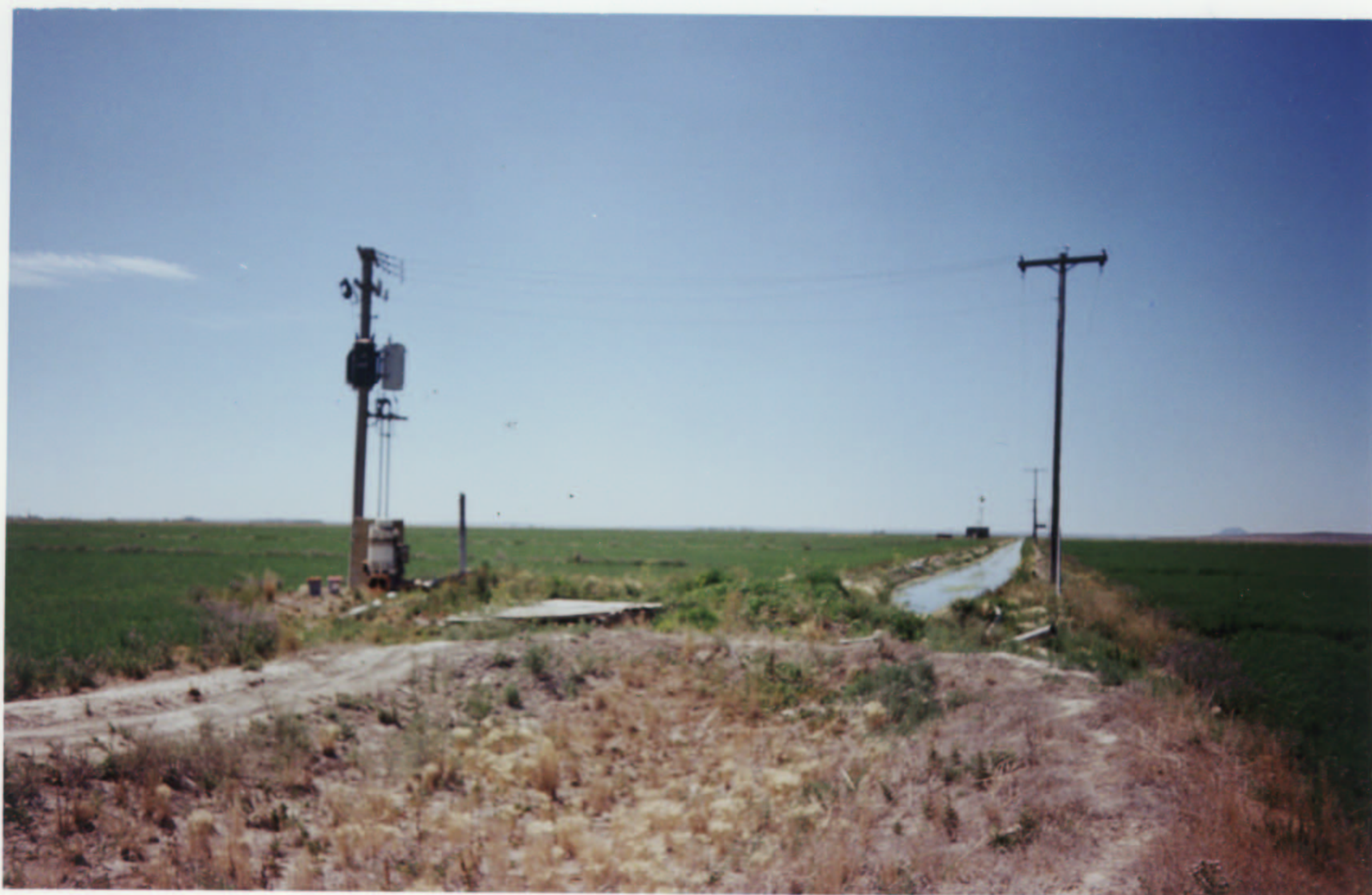
LOOKING SOUTH-SOUTH EAST AT WELL AND PUMP NEAREST THE COUNTY ROAD, APPROX 60' SOUTH OF THE COUNTY ROAD
