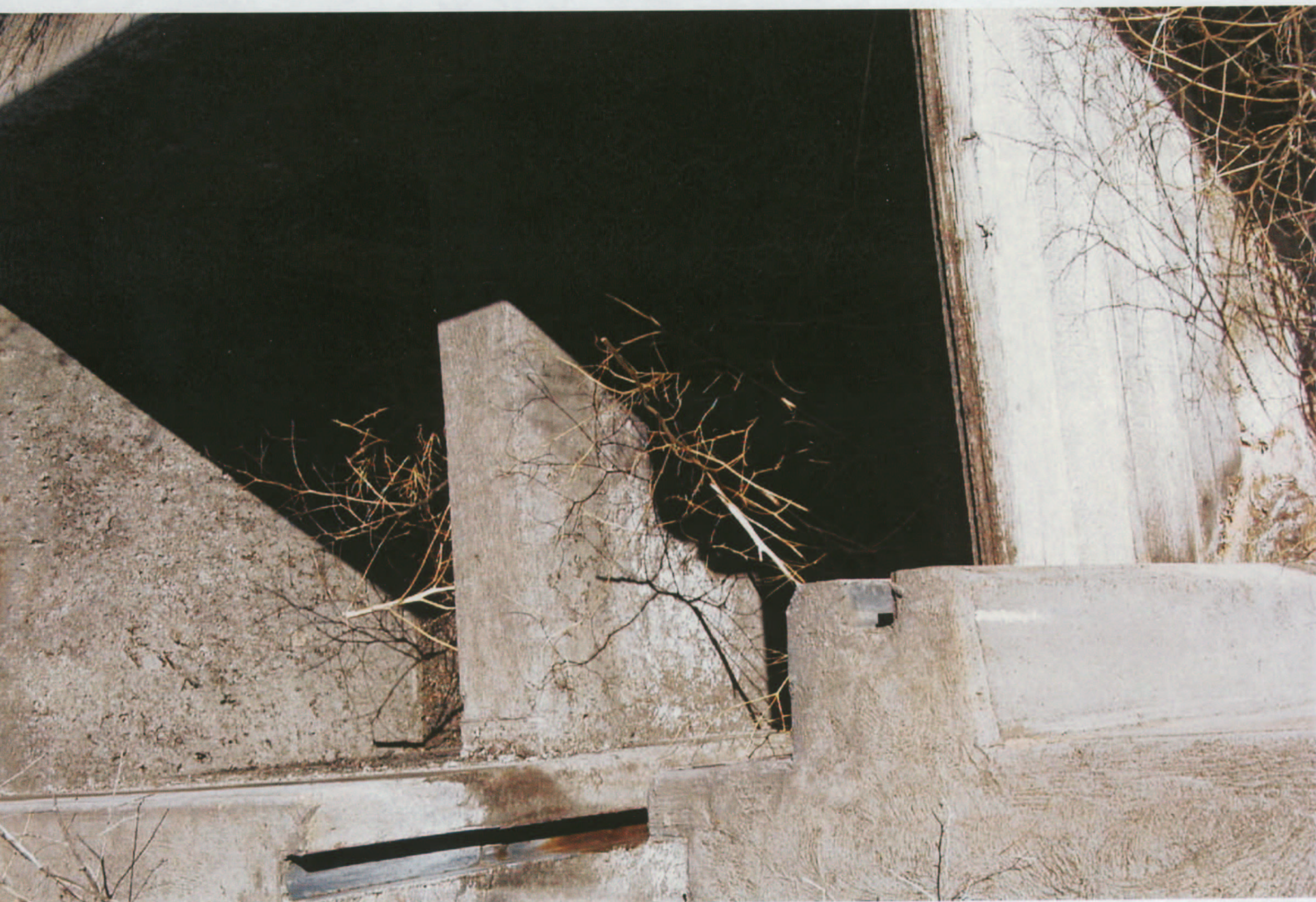
Looking down at diversion structure to raise water level in Camas Creek to allow flow East of Camas.
