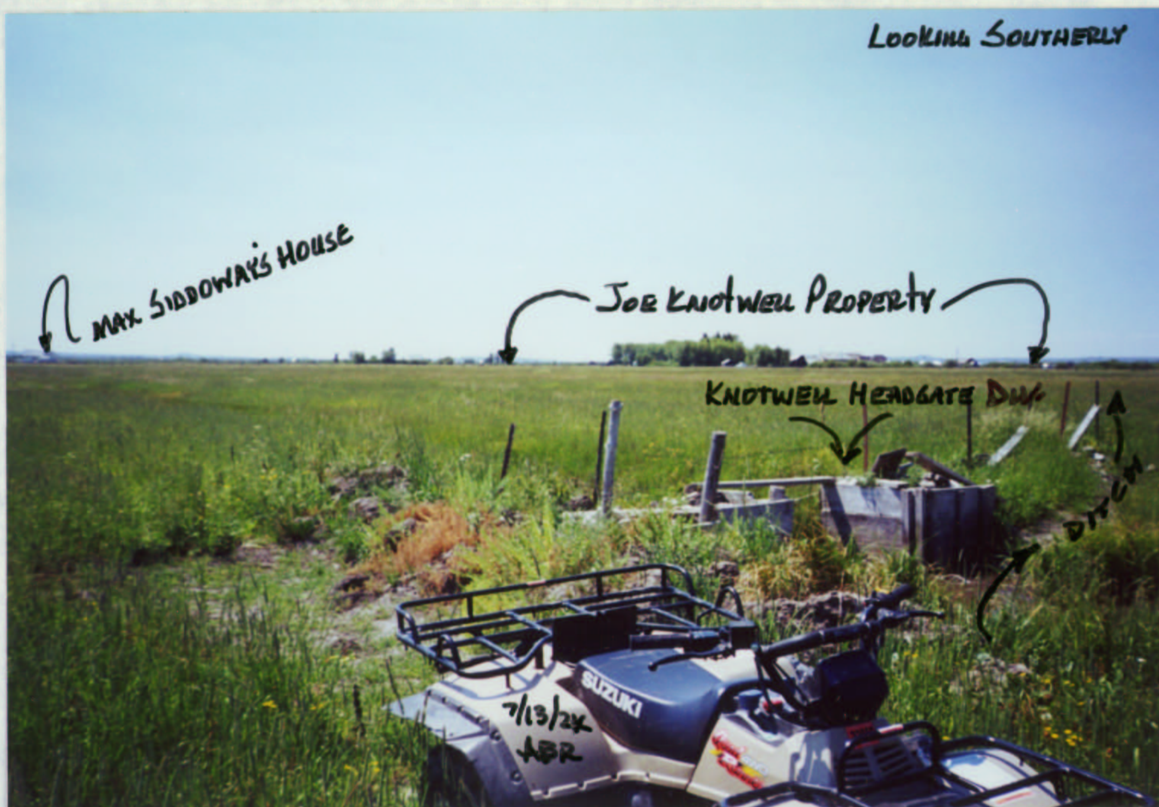
KNOTWELL'S FIELD HEADGATE IN SIDDOWAY'S FIELD.
