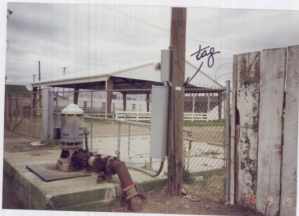
gps tag # A0002619 on power pole
