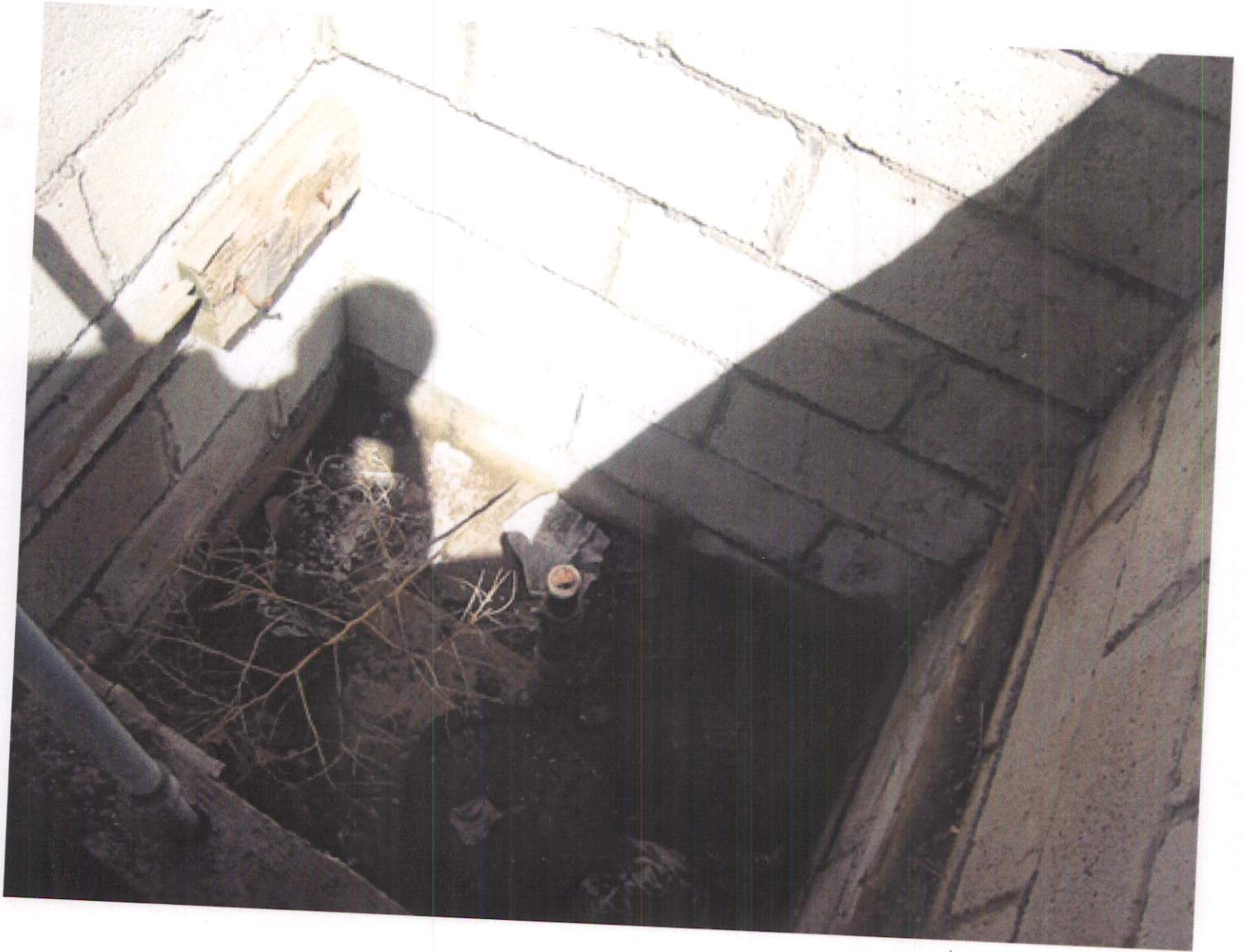
7/09/03 WPAJ. Hand-driven sandpoint w/ pump removed. Commercial well.
