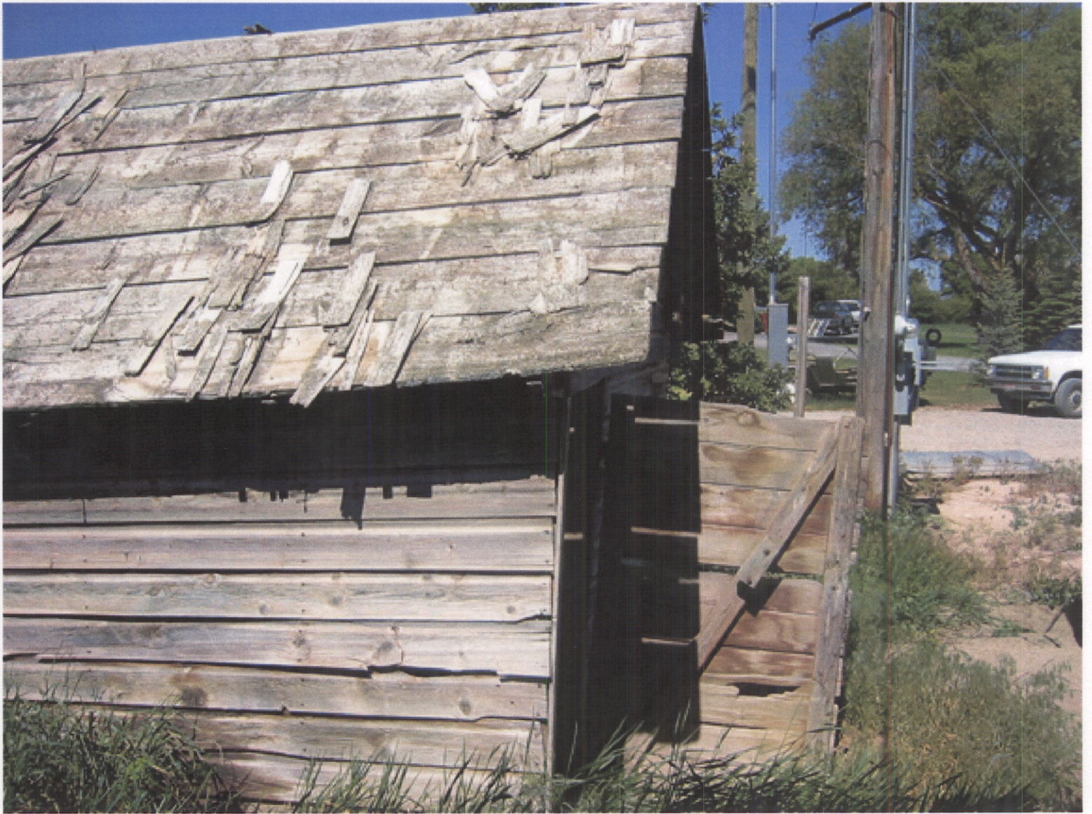
old shop used at time of original home. 6/10/2003
