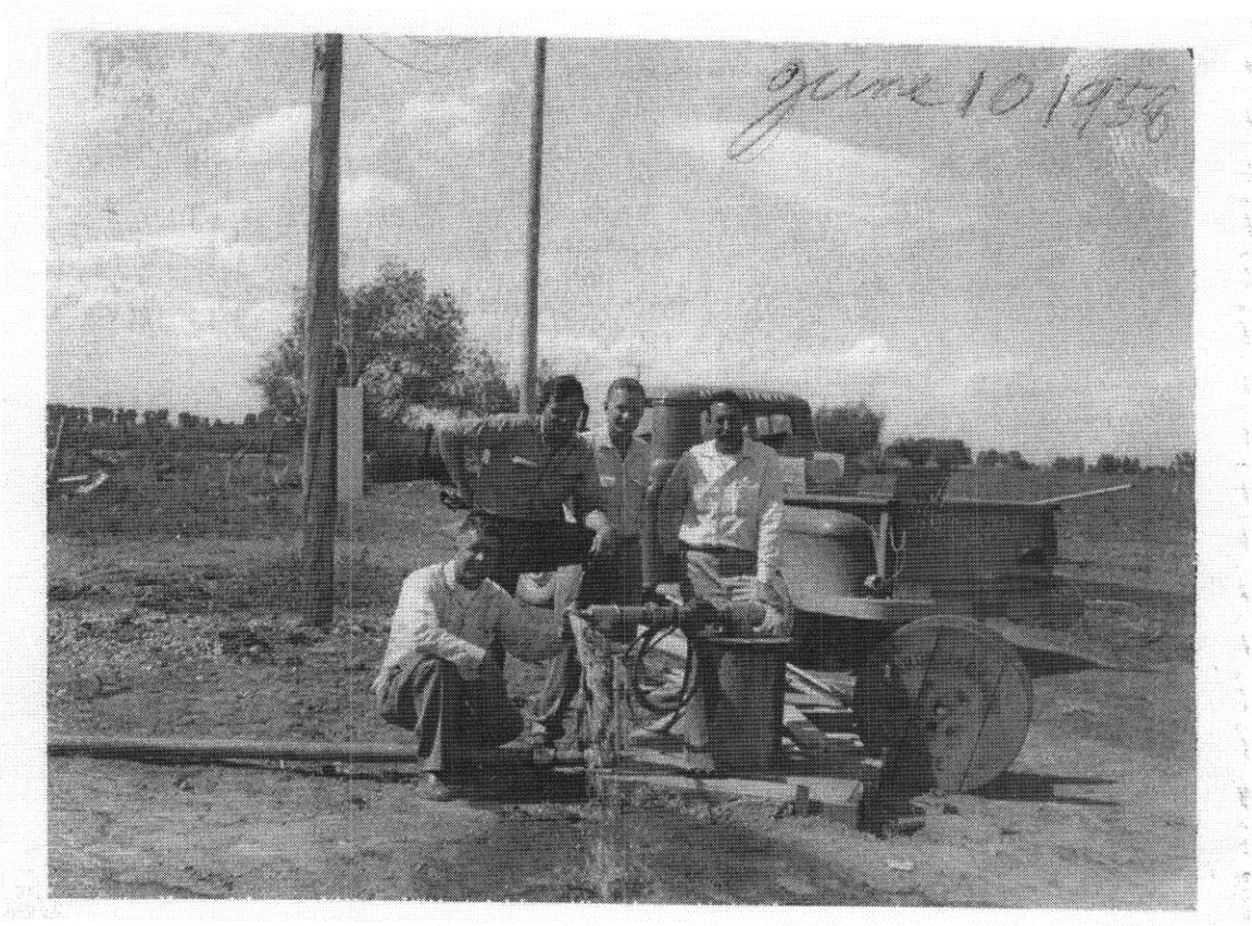
Falls Water Company, Inc. Completion of Well #1 Photograph Date: June 10, 1958 Source: Wilcox Construction Co Scrapbook
