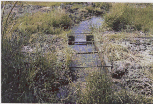
Weir below pond.
