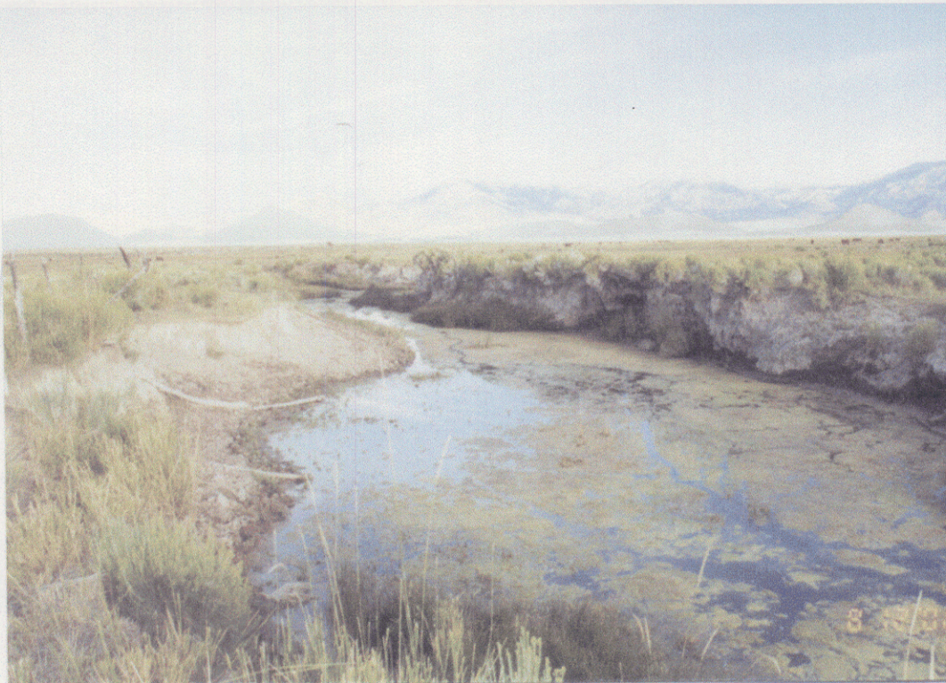
POINT #7 WEST OF EARTHEN DAM
