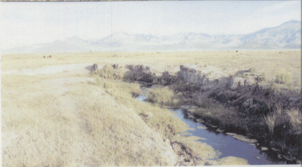
POINT #8 WEST OF EARTHEN DAM
