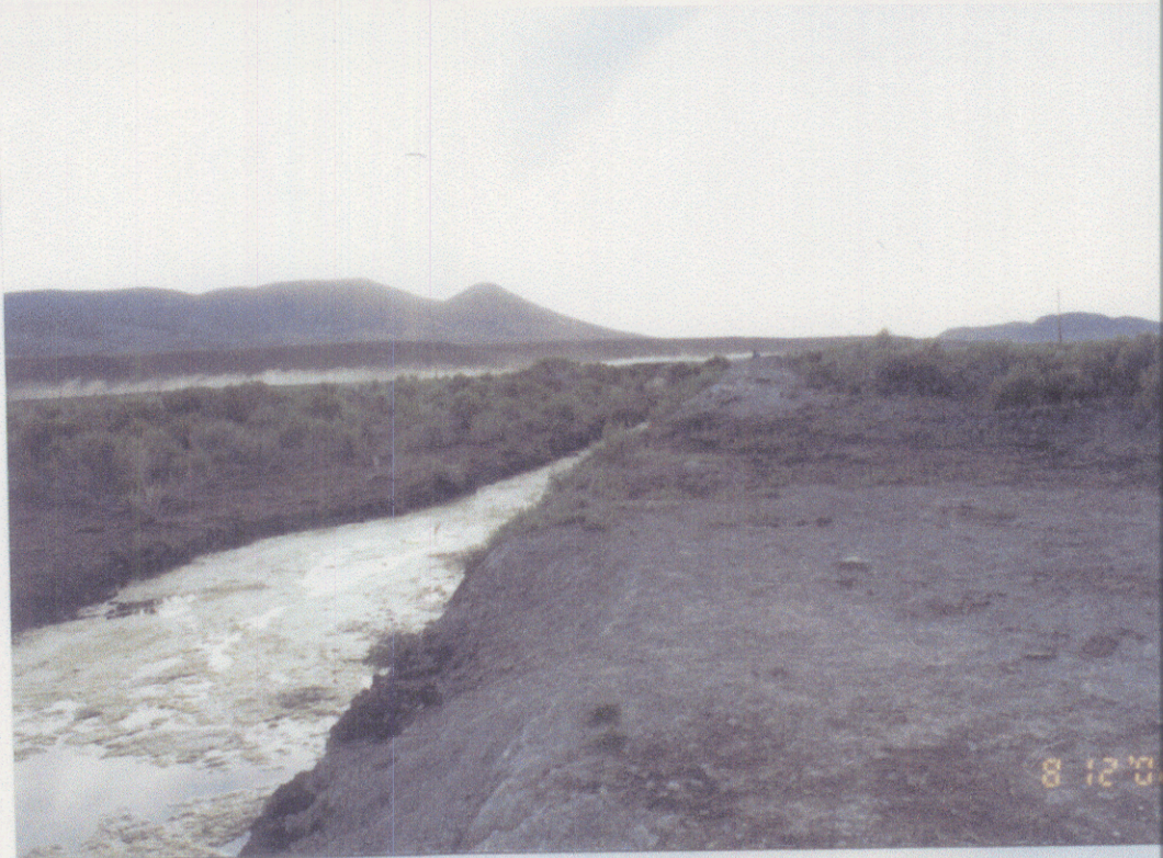
POINT #1 EARTHEN DAM LOOKING WEST EAST
