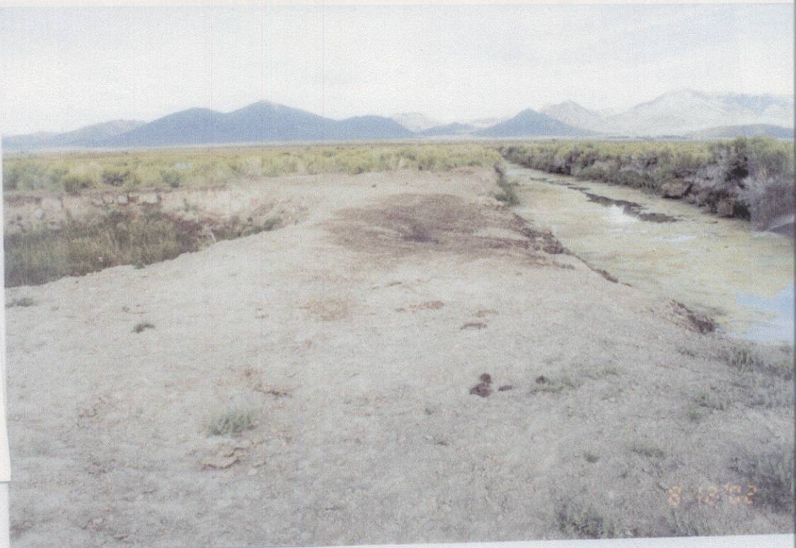
POINT #1 EARTHEN DAM LOOKING WEST
