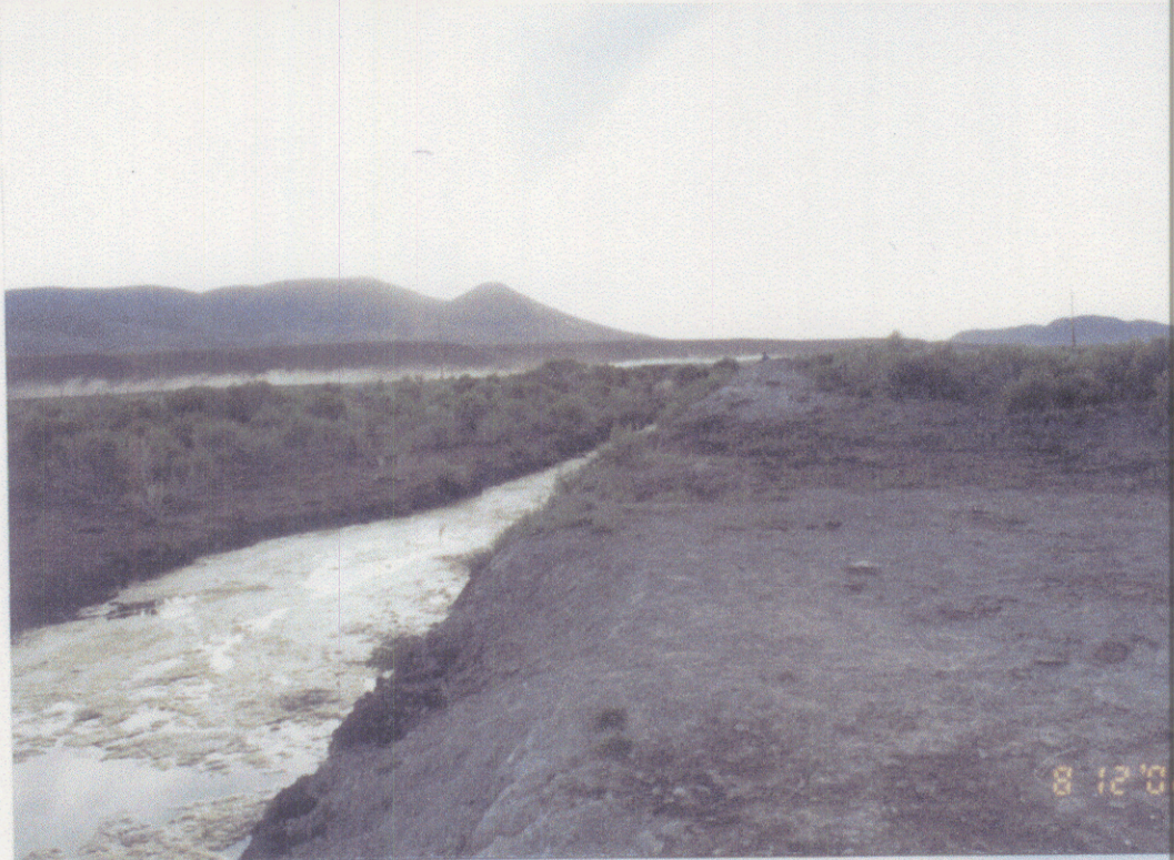
POINT #1 EARTHEN DAM LOOKING WEST EAST
