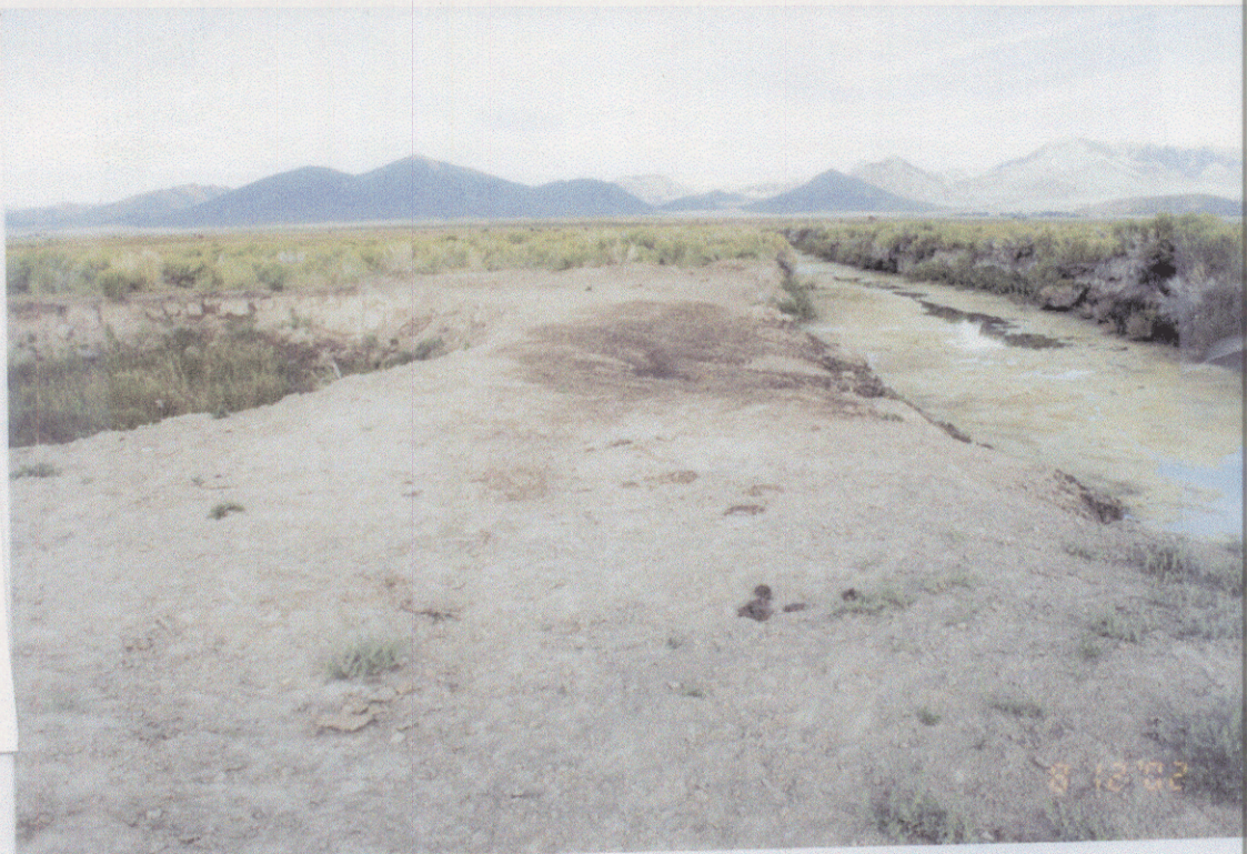
POINT #1 EARTHEN DAM LOOKING WEST
