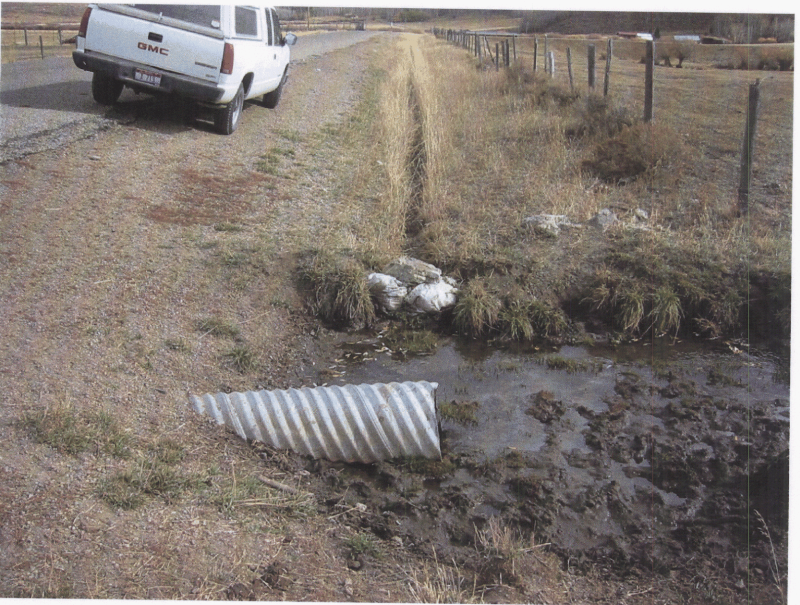
Second diversion from Gravel Creek- Ditch runs parallel to road while stream flows through culvert and under the road.
