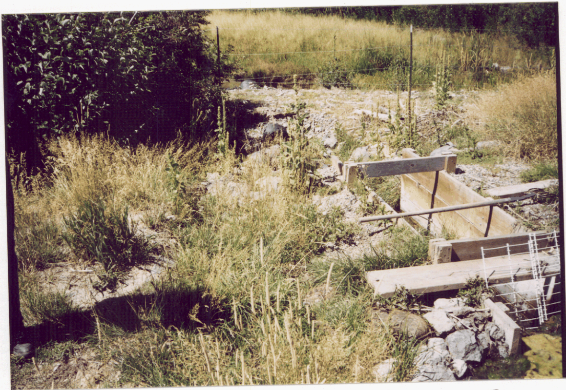
OUT LET For Irrigation Pond Stream go's To River
