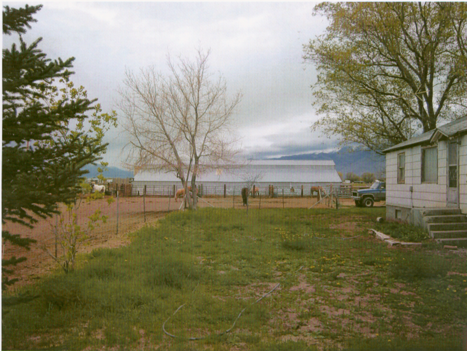
looking N from the front of the house
