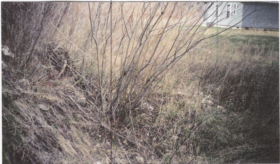
Photo 2. Shows A PLACE BEHIND THE BLOCKAGE OFF THE CREEK. OBVIOUSLY THERE HAS BEEN NO MAINTENANCE AND NO DELIVERY FOR A LONG TIME.
