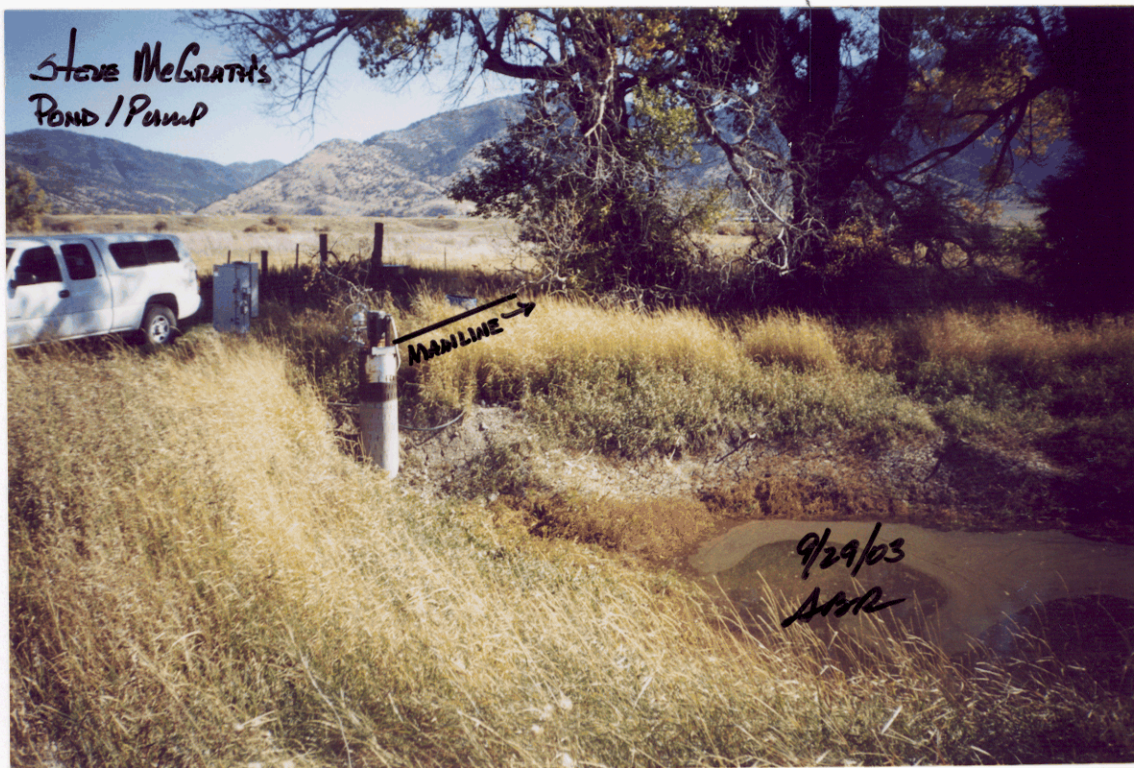
Photo 2. Shows POND, FROM E. END OF RAINEY CK., AND THE PUMP TO MAINLINE. MAINLINE ONLY GOES EAST.
