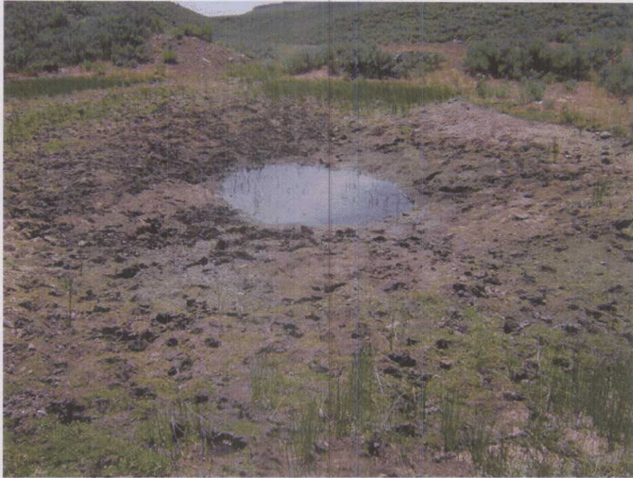
Minimal storage capacity due to partially washed out dam.
