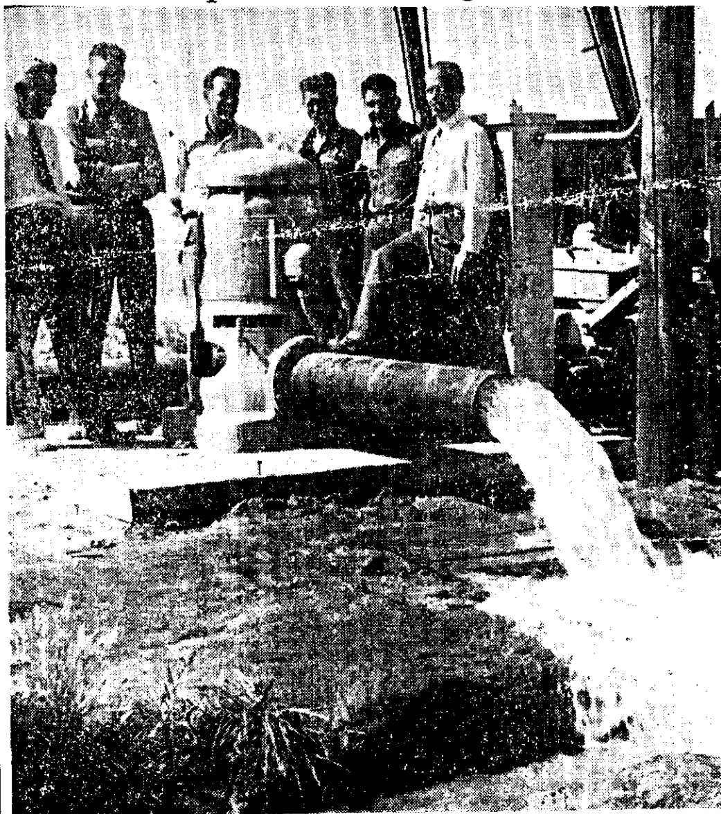
Water from an underground stream 250 feet below the surface of the C. W. Colner ranch near Hansen is shown above flowing from a new 75-horsepower turbine pump installed Saturday. Men who helped install the pump are pictured left to right inspecting the test flow of water. They are J. B. Wade, Peerless pump engineer; Paul Neumann, Henry Colner, Alfred Carlson, Jack Witherspoon and Emery Gard. Water is flowing from a 16-inch pipe. (Kelker photo-staff engraving)
