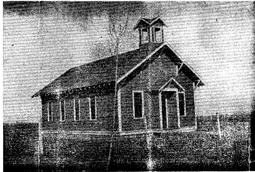
CLOVER LUTHERAN AROUND 1915 — This building served as both a school and a church for the Clover Lutheran congregation until 1918 when the present church was built. (Photo courtesy of Orval Reinke.)
