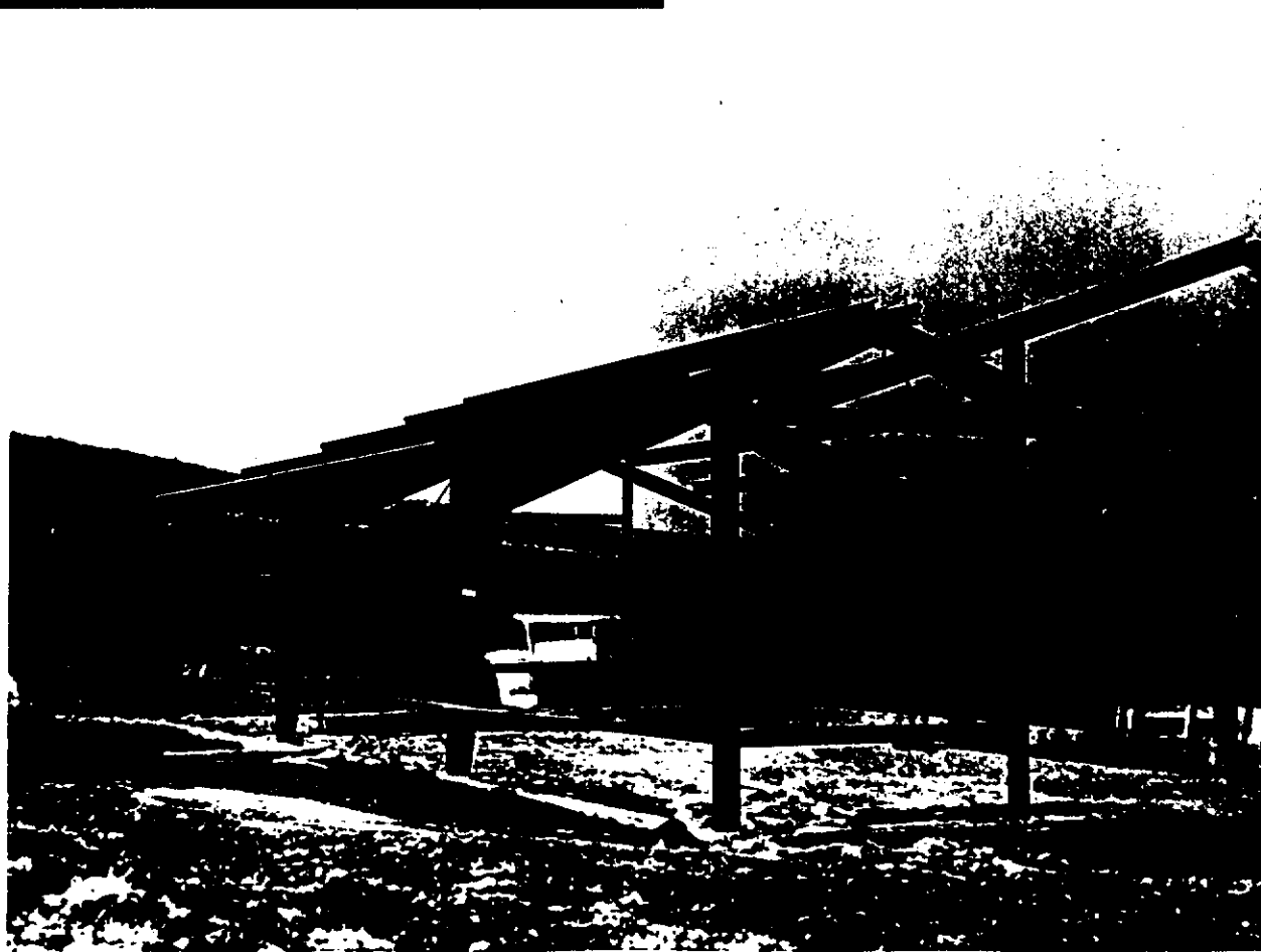
Framework and foundation of our steel building at Grays Lake Refuge.
