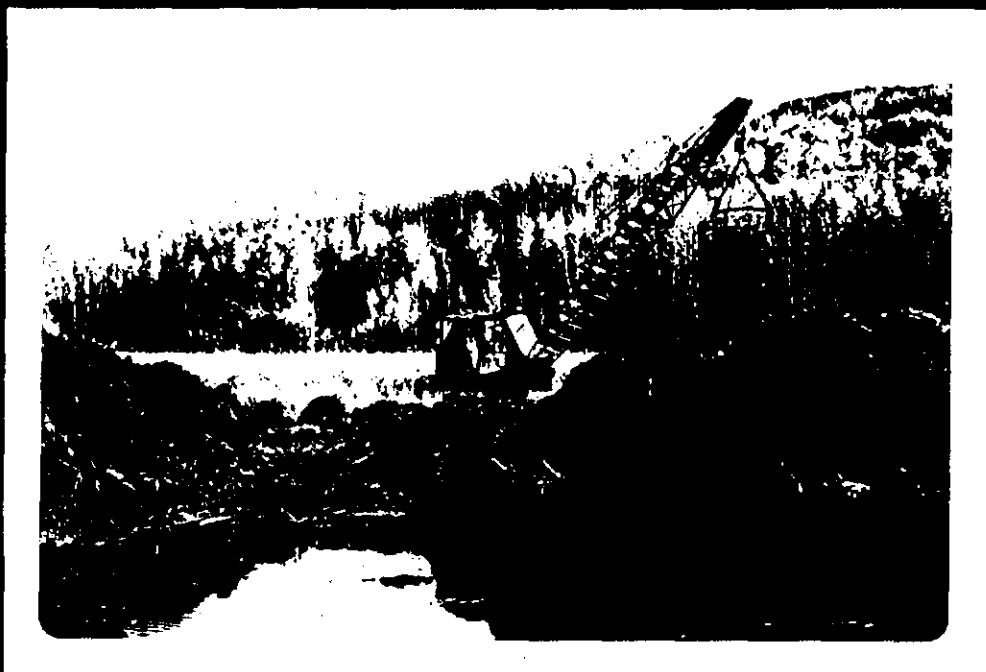
The Schield Bantam Dragline used by contractor to dig potholes at Grays Lake proved highly suitable for marsh work. Its light weight and wide track enabled it to work with great efficiency.
