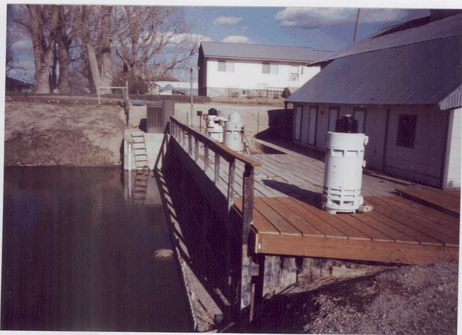
Mud Lake Water Users Main Pumping Station, 6N 34E 24 NENE.
