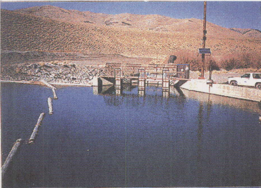
Photo 1. INTAKE FOR THE DRY CREEK HYDROPOWER AQUADUCT. ALSO SERVES AS THE POINT OF DIVERSION FOR SEVERAL DECREED RIGHTS FROM DRY CREEK. THESE RIGHTS ARE NOW DELIVERED AS DEVELOPED WATER AHEAD OF AND OUT OF SEQUENCE OF OTHER DECREED RIGHTS OF THE LITTLE LOST RIVER SYSTEM.
